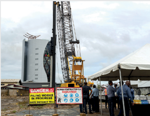
Driving of the first pile of Tower B
